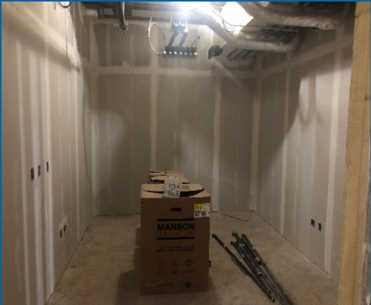
Admin Addition Drywall Hang/Tape/Finish
