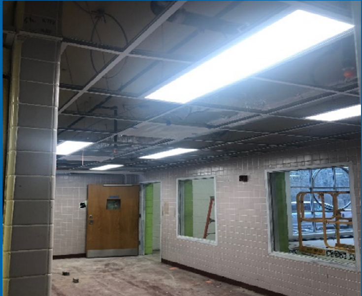
Kitchen Ceiling Grid and Lighting
