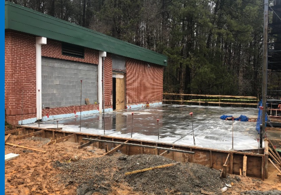
Classroom Addition Slab on Grade
