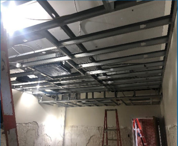
East Wing Hard Ceiling Framing
